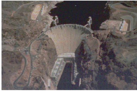
Hoover Dam is considered one of the greatest engineering works of all time.
